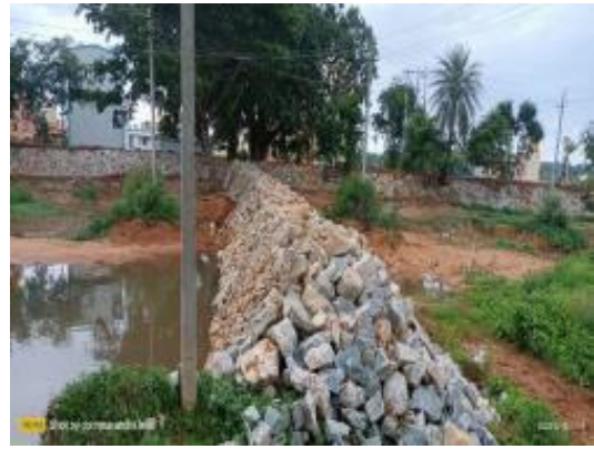
Stone built around sedimentation pond.
