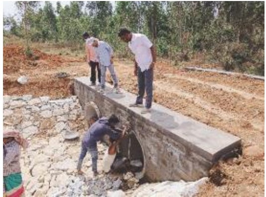
Completed inlet construction.
